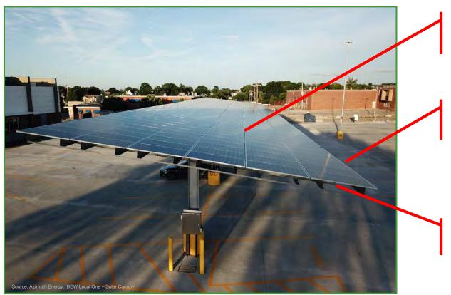
CANOPIES WILL NOT HAVE METAL DECKING (EXPECT PRECIPITATION TO DRIP THROUGH MODULE GAPS)
